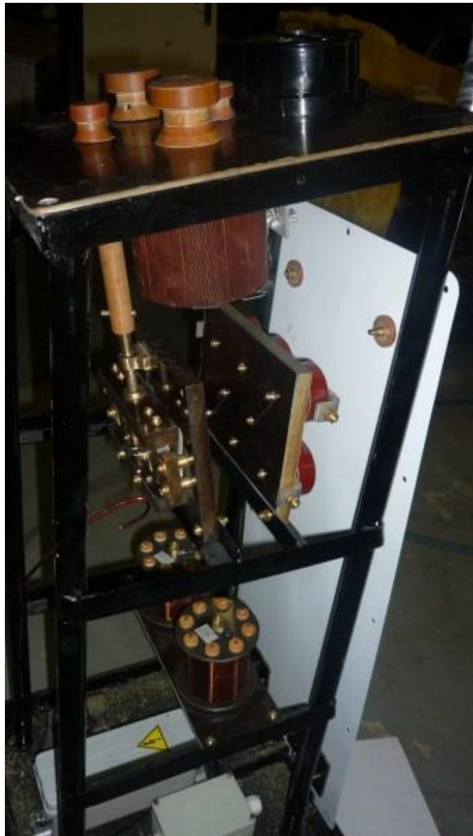
Final fitting of the key components ahead of wiring.
